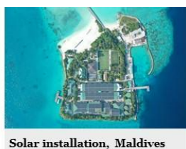
Solar installation, Maldives
