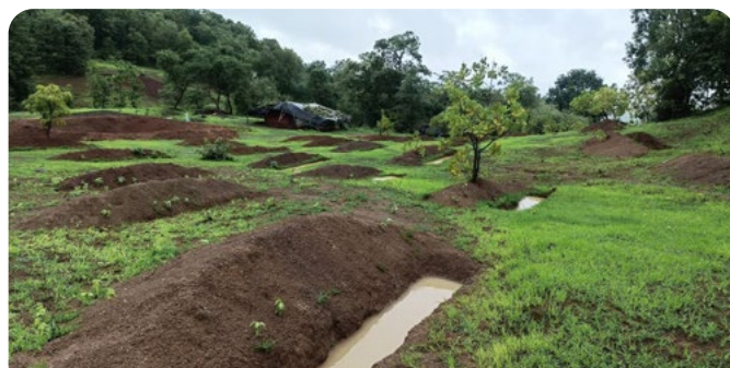
Continuous Contour Trenches dug along hill slopes
