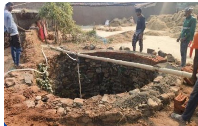
Identification of wells in want of restoration
