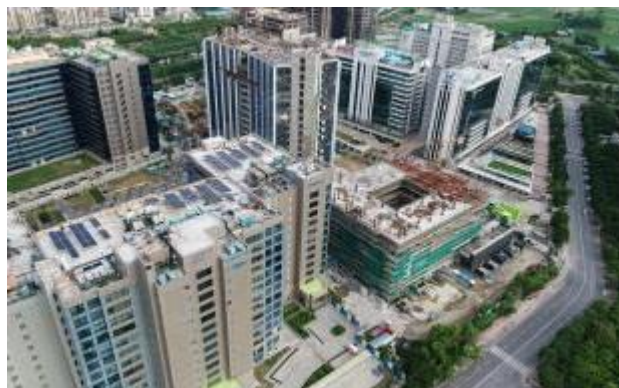
Tower 11 A (as of September 2020)
