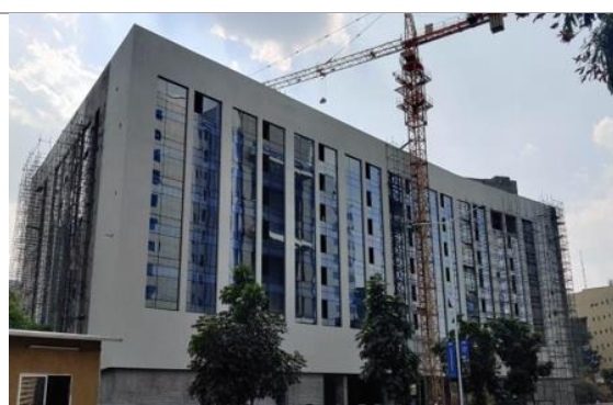
B-22 (Hotel): Structure Completed
